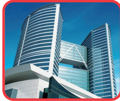
Albion Valves facility in the Jebel Ali Freezone
